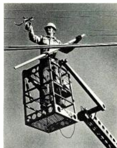
Hang it up. A Cablecom-General technician strings the Joplin fiber-optic cable.
